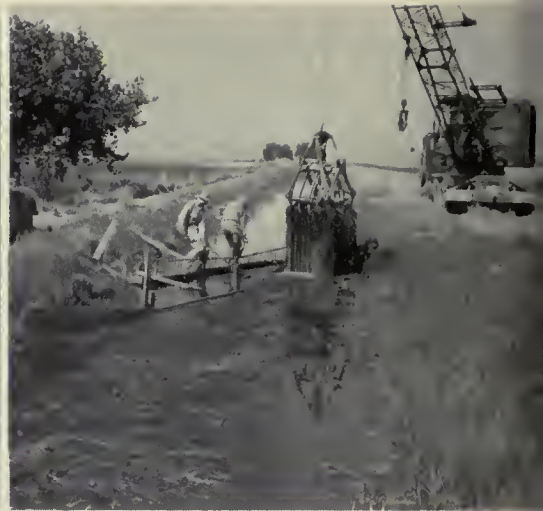
"MOSS FORK" in a close-up just before it is dropped into the water. At right, truck dropline in operation lifting weeds from loter as they float into homemade guide. The trap in these photos is the one previously used. Photos by A. M. Bergloff, Region
